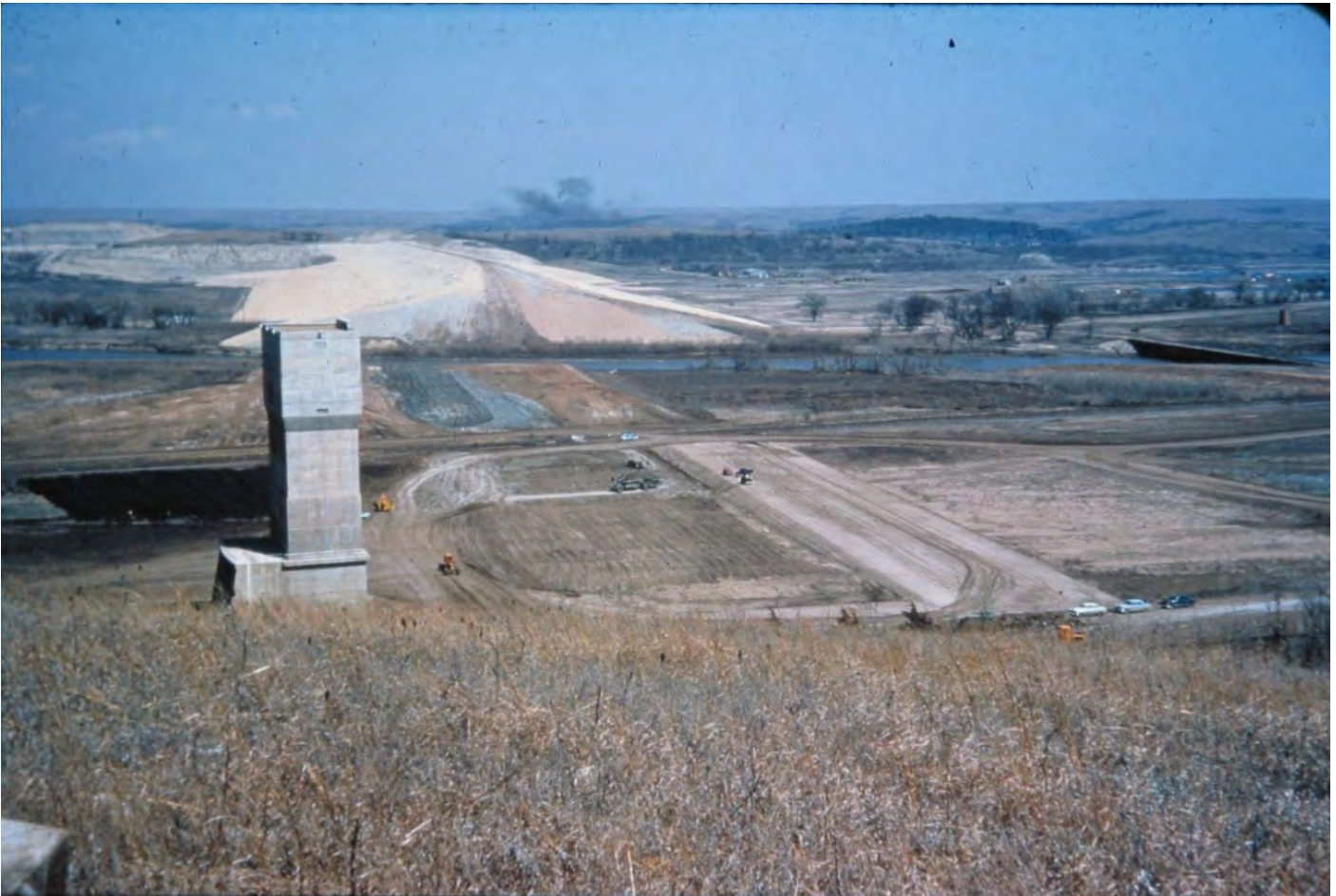
Tuttle Creek Dam north of Manhattan under construction. About 1958. Photo courtesy of Roy Bird.
