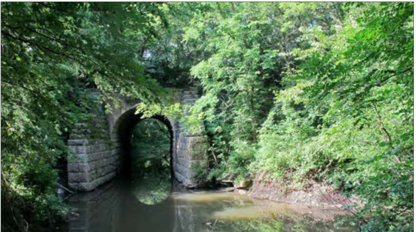
An old, abandoned railroad bridge near the present town of Bala, Kansas. Photo taken in 2014 by Judy Regehr.
