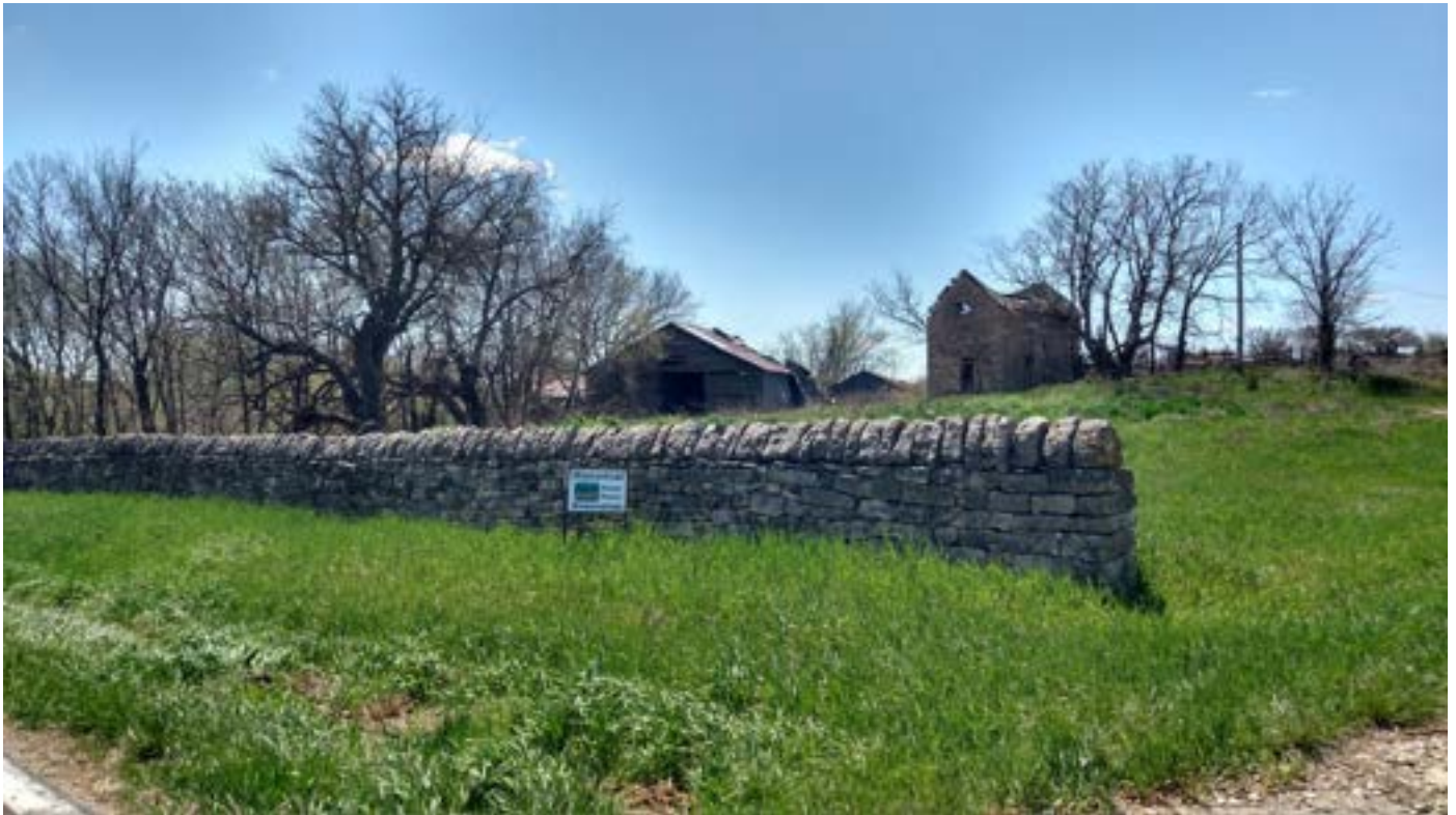
Highway 99 stone fence
