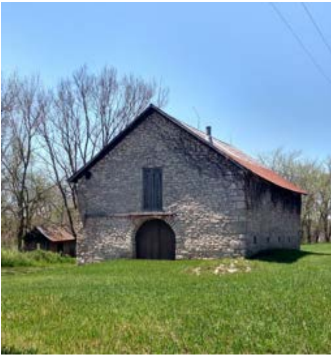
Stone barn outside Dover, heading to Eskridge
