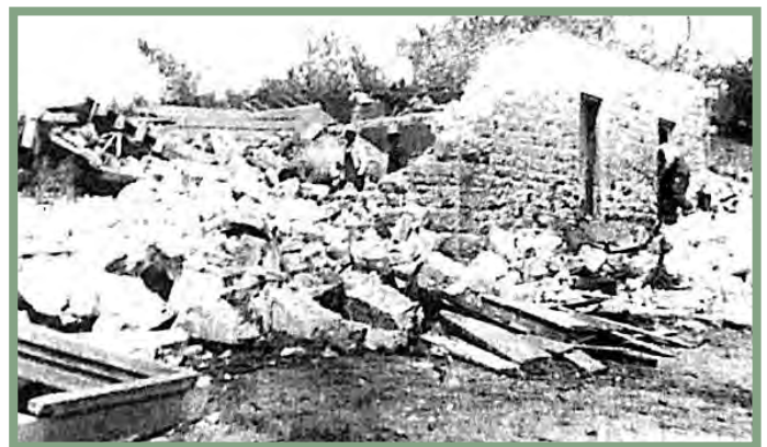
Blasing Springs Hotel after it was hit by a tornado on May 15, 1943. Source: Winifred Slagg, 110
